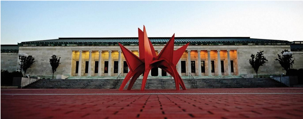
Figure 7. Toledo Museum of Art main building (Greek ionic façade), http://www.toledomuseum.org/
